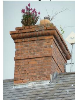
View of foliage growth, perished pointing and spalled brickwork to the rear chimneystack
