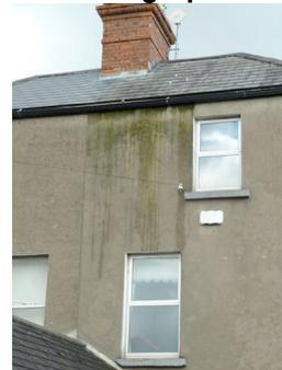
View of damp staining to the rear elevation
