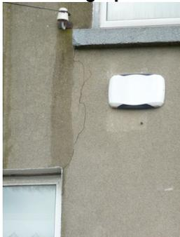
View of cracking to the rear elevation
